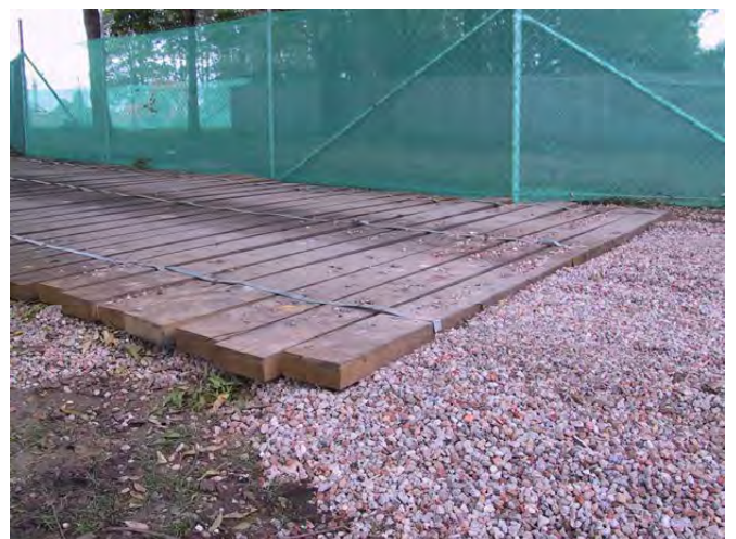
Figure 5.4 - Example of proper ground protection when access is required through a Tree Protection Zone (TPZ).
