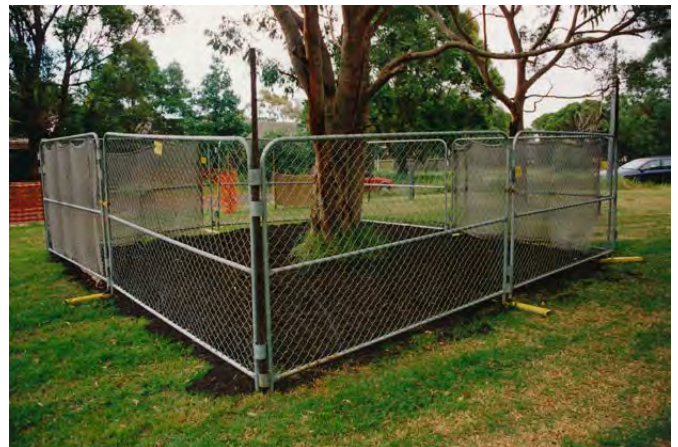
Figure 5.3 - Example of proper tree protection fencing used to define and protect the area around a tree.
