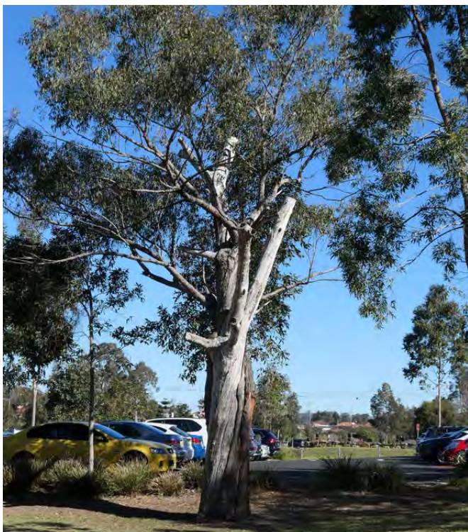
Figure 7.4 - At some point, all trees will reach the end of their useful life and require removal.
