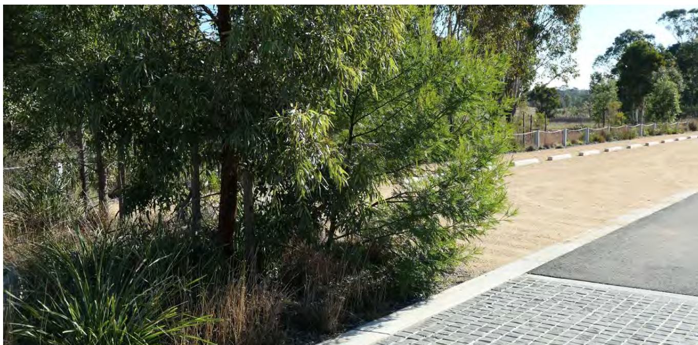
Figure 3.12 - Trees that are low branching and planted too close to roads and car parks can present a safety issue, particularly when near pedestrian crossings. These trees need to be appropriately managed to maintain adequate sight-lines between pedestrians vehicles and to signage.
