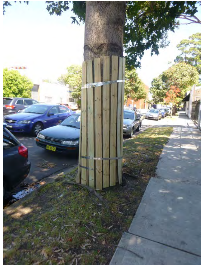
Figure 5.5 - Example of proper trunk protection when work is required in very close proximity to a tree.
