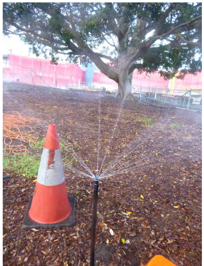
Figure 5.6 - It is often advisable to insist on temporary irrigation around significant trees to ensure they remain in optimum health while work is undertaken in close proximity or where some roots are likely to be impacted due to proposed works.
