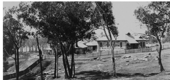
Image taken from South of buildings showing the Convalescent Cottages prior to extensions. c1903. Mitchell Library, State Library of New South Wales
